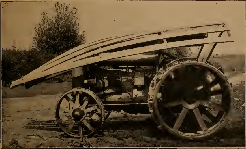
FIG. 16. Fordson tractor equipped with a shield for orchard work, designed by E. L. Main, Delaware, O. The boards, being smooth, lifted the limbs without injury.
